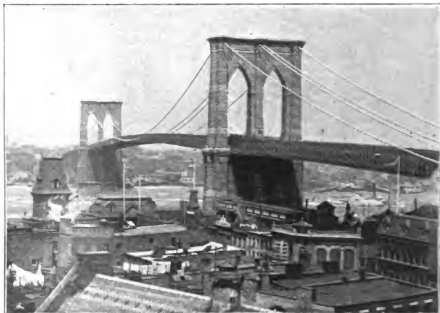
EAST RIVER BRIDGE, FROM NEAR THE BROOKLYN LANDING.
